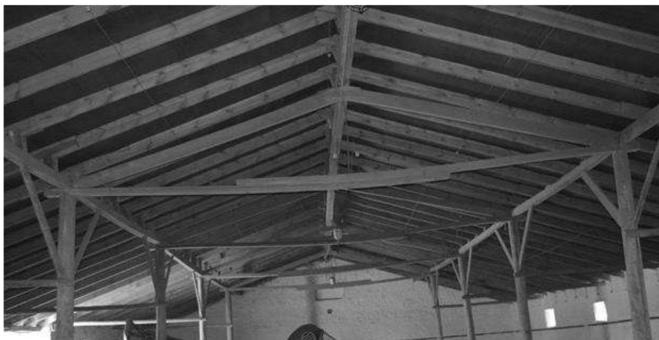
Fig. 1. Internal load-bearing wooden structures of grain warehouse No2
